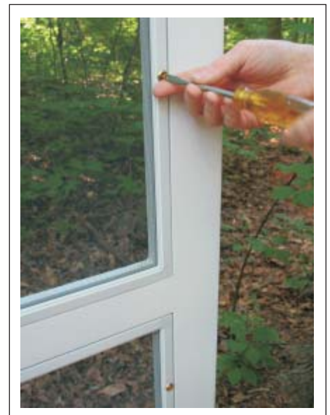
Two removable panels sit in a rabbet, flush with the inside of the door, dividing at the middle rail. They are easily removed with a flat head screwdriver. The aluminum screen and storm frames are available in white or dark bronze.
