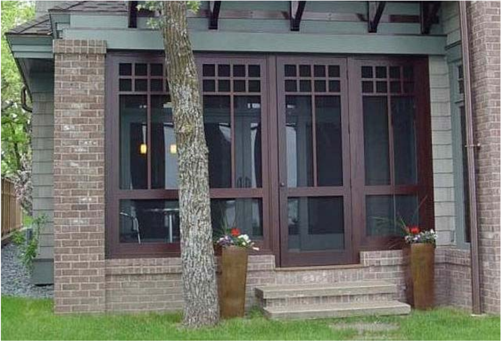
Three season porch with Touchstone Woodworks' Craftsman style mahogany door and wall panels with Sikkens Dark Oak finish.
