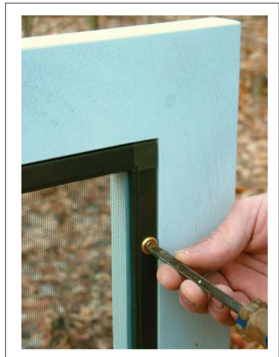
The removable panel sits in a rabbet, flush with the inside of the knee wall panel. They are easily removed with a flat head screwdriver. The aluminum screen and storm frames are available in white or dark bronze.
