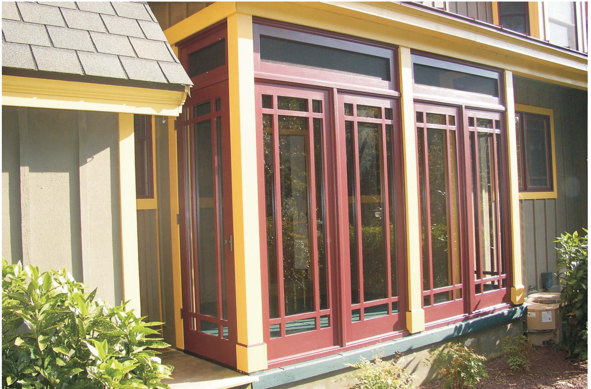
Three Season Porch Touchstone Woodworks' Prairie View Wall Panels and single lite transoms
